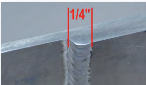
Weld Must Be 1/4 Inch Wide
